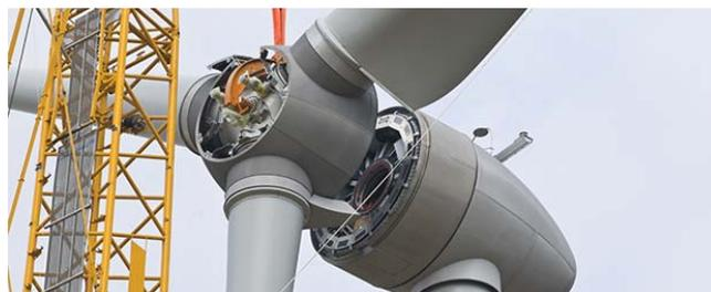
Figure 3. WT bearing replacement, [16].
