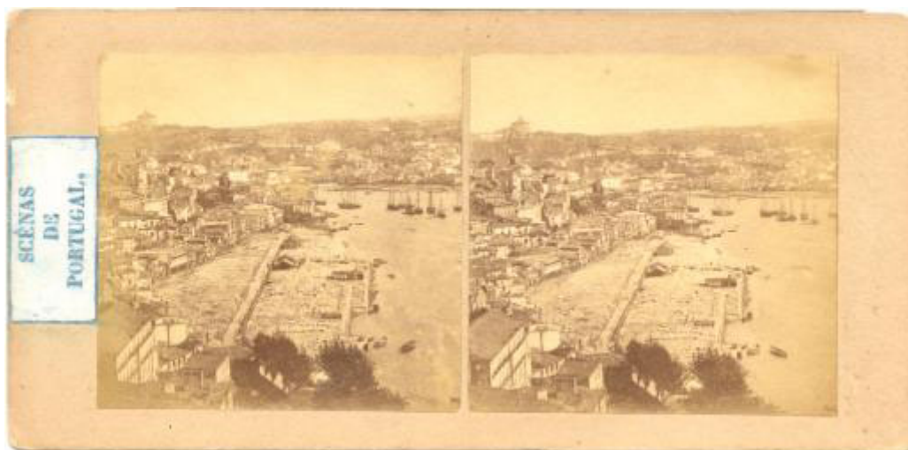
nn9 - Construction of the New Customs House (Alfândega Nova) - (courtesy of Alexandre Ramires)
