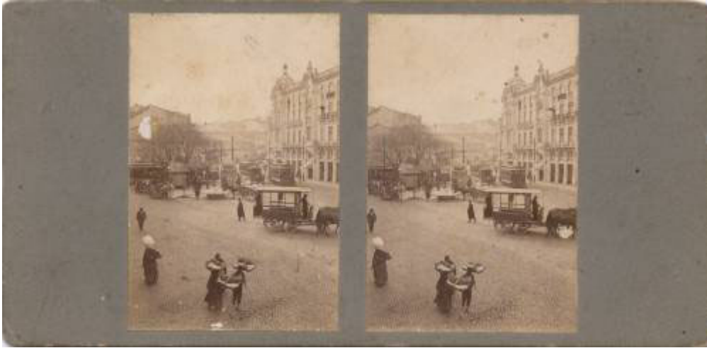
nn9 - (view of the Intendente square) - Nice example of a late stereoview (probably early 1900s), with occupational (fish sellers) and transportation (electric tramway, animal traction) interest.
