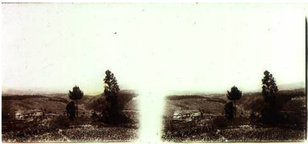
nn1 - Wide view of a rural property -
