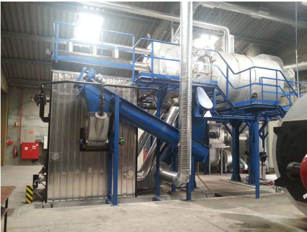
Fig. 4. Biomass system in a textile dyeing plant in north Portugal – steam boiler.
