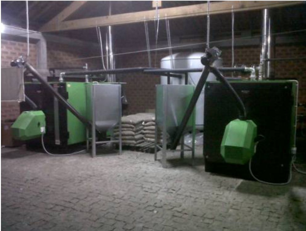
Fig. 1. Example of a heating system in an elderly care centre in north Portugal, composed of two 150 kW th boilers.
