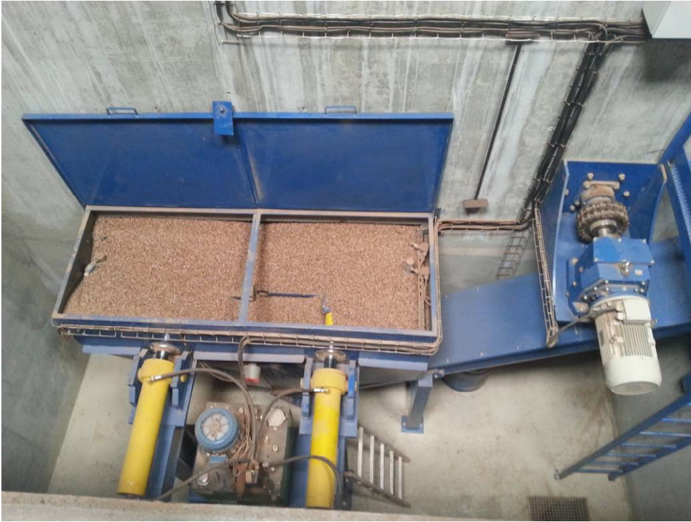
Fig. 3. Biomass system in a textile dyeing plant in north Portugal –wood pellet feeding.
