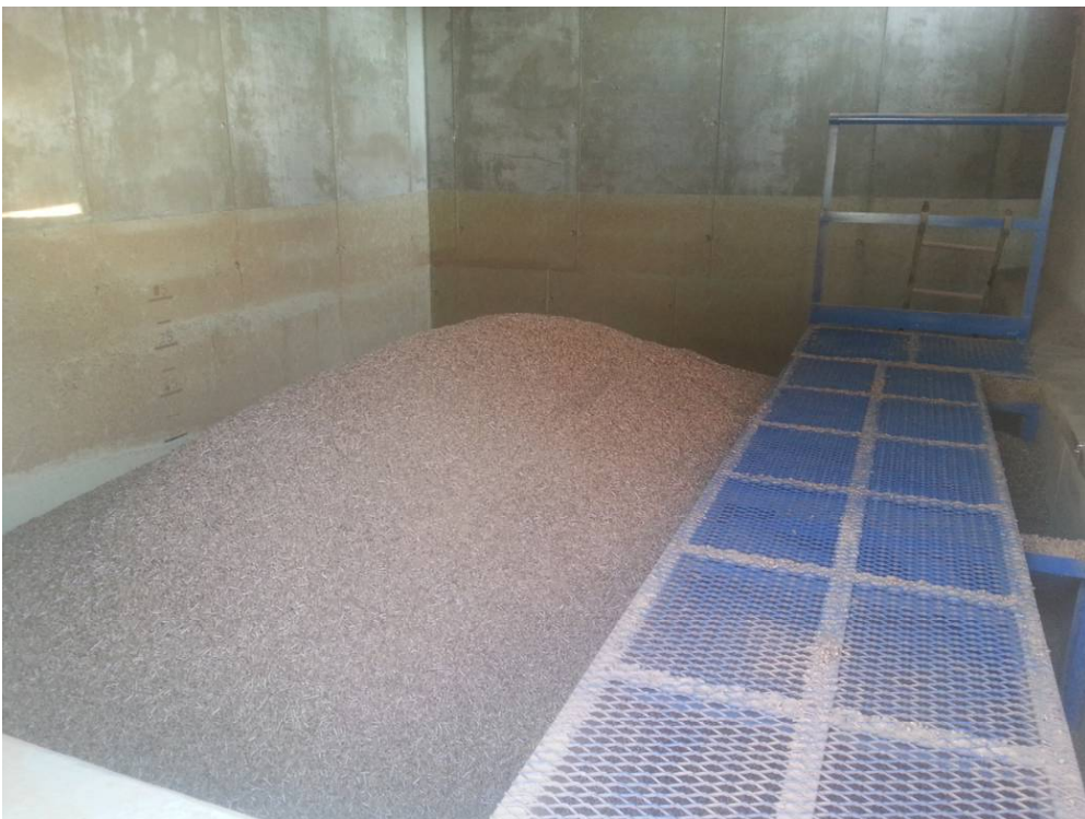
Fig. 2. Biomass system in a textile dyeing plant in north Portugal –wood pellet storage.
