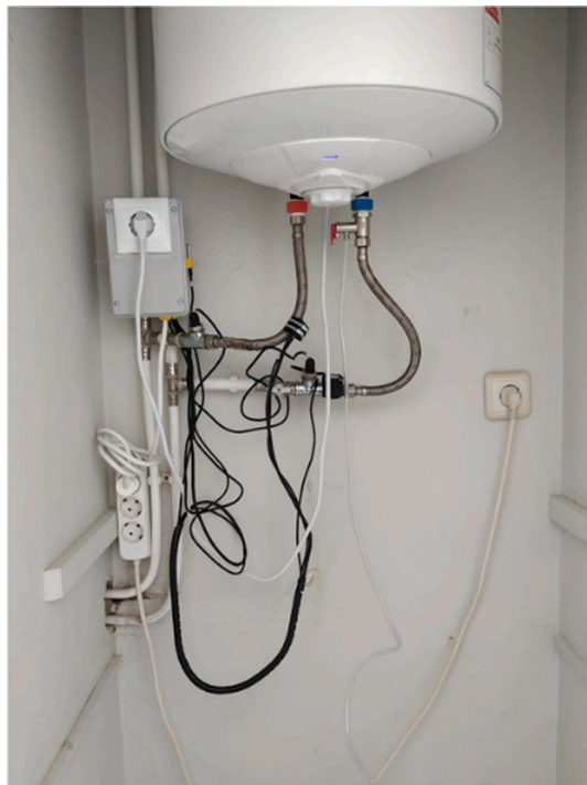
Fig. 10. Typical installation of a Klugit device.
