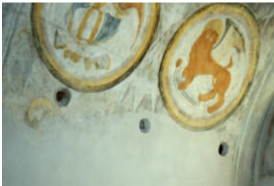
Figure 1 and 2: Acoustic pots openings at Villette church and one of its pots (found in 1927 and now in a Museum).
