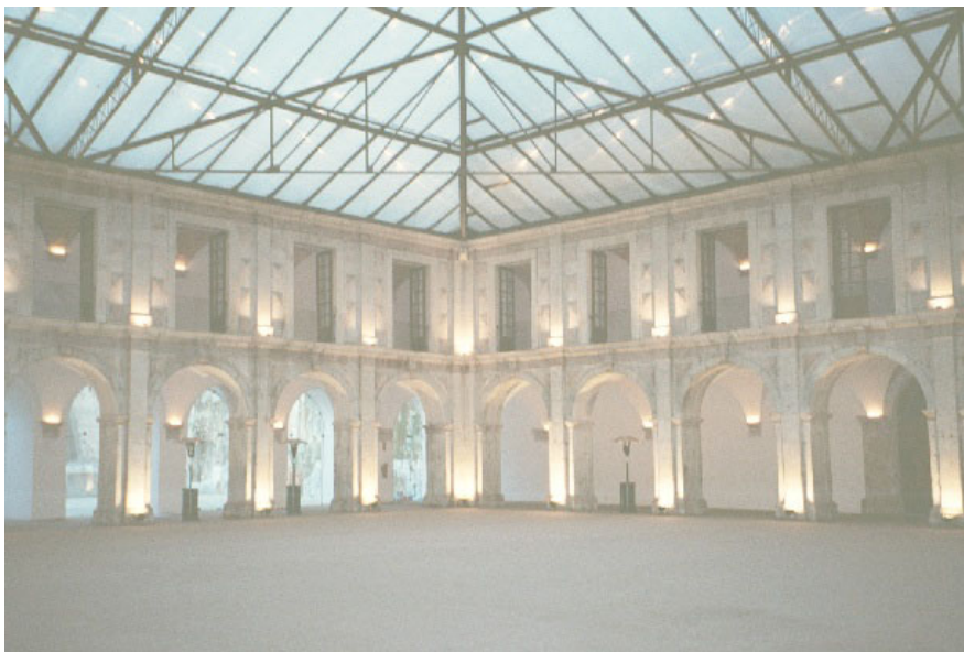
Figure 16: Photo of cloister CB (Beato Convent) with specific particularity (closed patio).
