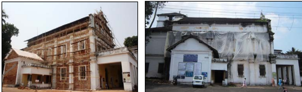
Figure 1. Nossa Senhora do Pilar church (Goa, India) during and before restoration.
