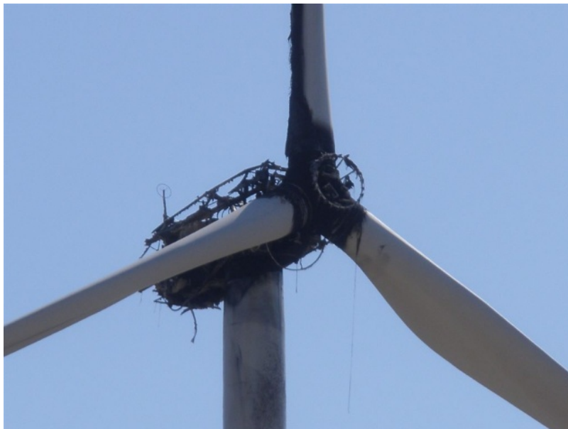
Fig. 2. Wind turbine in Portugal damaged by lightning.
