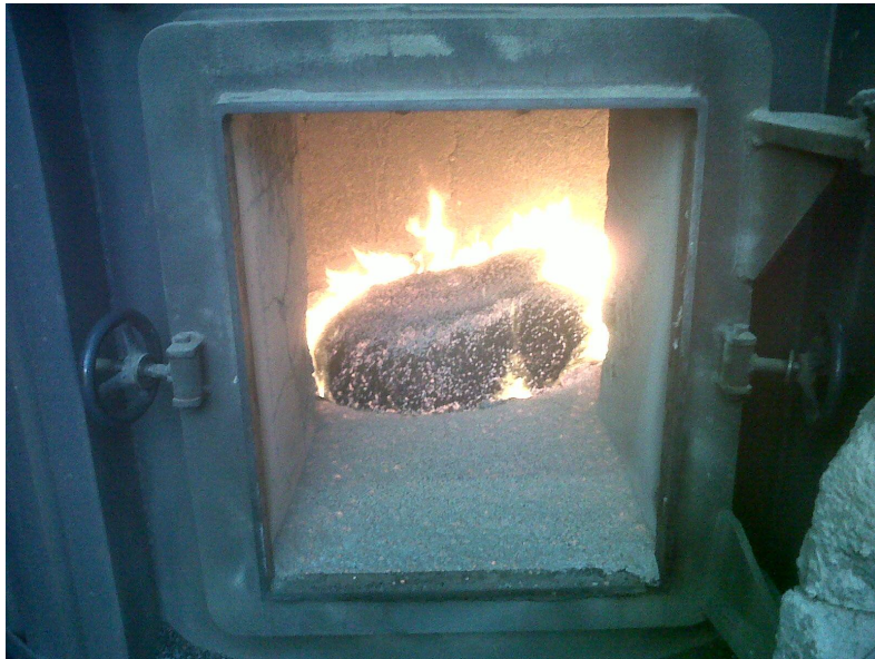
Fig. 1. Ash formation over a furnace grate fuelled with wood pellets.
