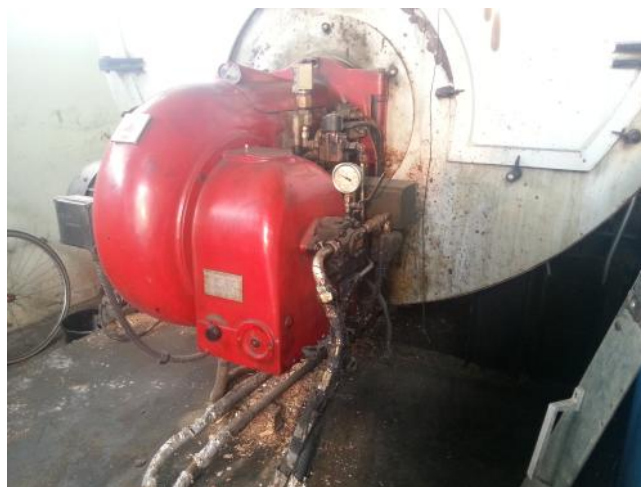
Fig. 3. Naphtha burner in a steam boiler.
