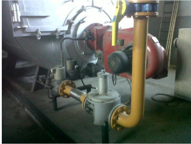
Fig. 1. Natural gas burner in a steam boiler.
