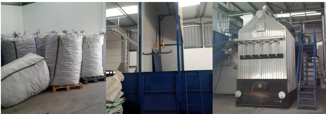
Figure 6. Warehouse storing big-bags with cotton briquettes; silo furnace loading system; the steam boiler furnace.
