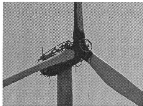
Fig. 9. Wind turbine in Portugal damaged by lightning
